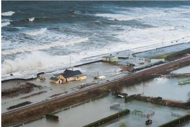
Figure 1. Coastal flooding experience during the January 2014 storms (© Mike Alexander, 2018)
