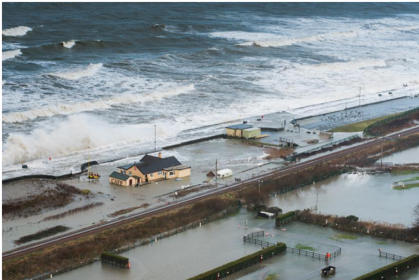
Figure 16. Coastal flooding experience during the January 2014 storms (© Mike Alexander, 2018)
