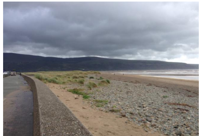
Figure 13. Sand dune system protecting the southern end of the promenade from wave action (Arup, 2018)
