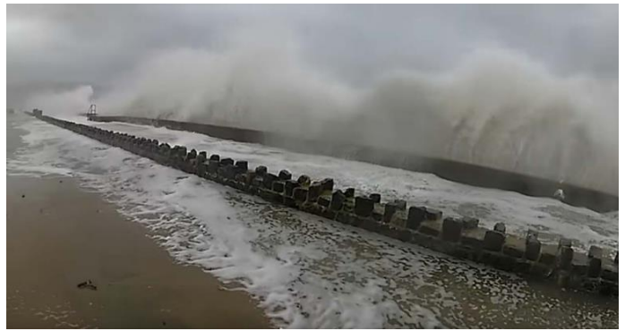
Figure 15. Wave overtopping at North Barmouth during Storm Brian (21 st October 2017) (Image: youtu.be/gVtJ8t7T7uQ )
