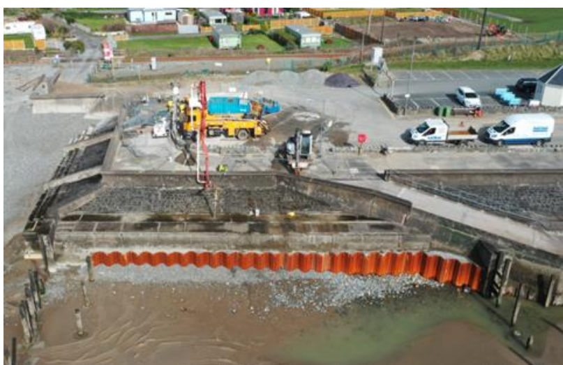
Figure 23 Emergency repairs in April 2021
