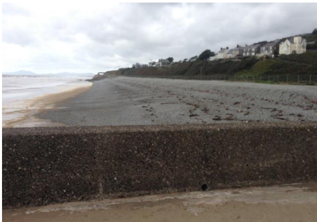
Figure 12. Shingle berm providing protection to the railway line at the north of the promenade (Arup, 2018)
