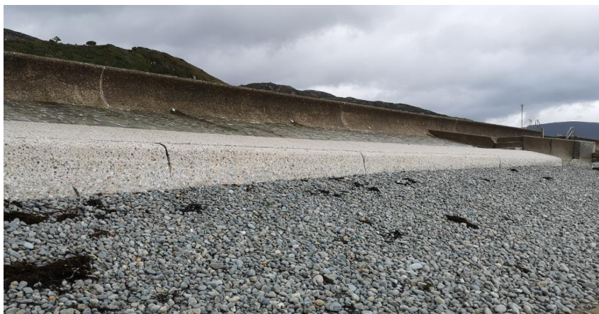
Figure 10. The concrete wave recurve wall with shingle foreshore at southern end (Arup, 2018)
