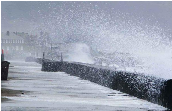
Figure 14. Overtopping of promenade at Barmouth in 10 th December 2014 (Image: Daily Post Wales)
