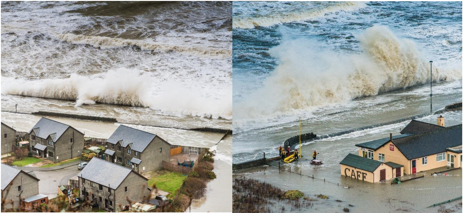
Overtopping and coastal flooding experienced at Barmouth North Promenade in January 2014 (images copyright: Mike Alexander)
