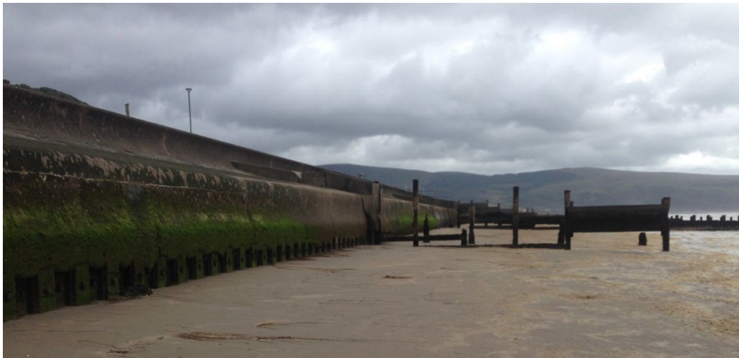
Figure 35. Defence of North Barmouth showing wave return wall, exposed sheet piling and groynes missing timber planks
